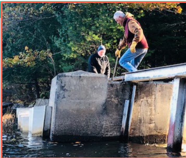
October 24: Dean Sciaraffa and Paul Crockett remove a board from the dam, lowering the lake six inches – Photo by Paul Fontaine
