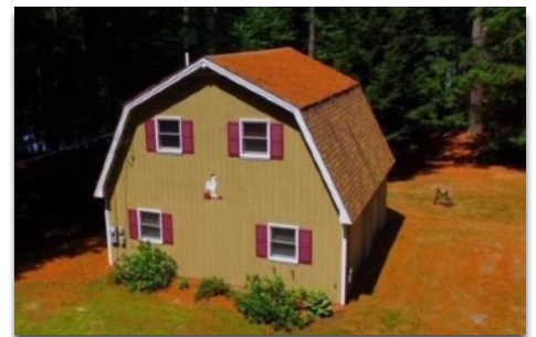
Garage Apartment - BEFORE
